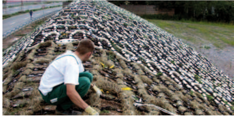
Extra coarse geotextile grids for erosion control on embankments
