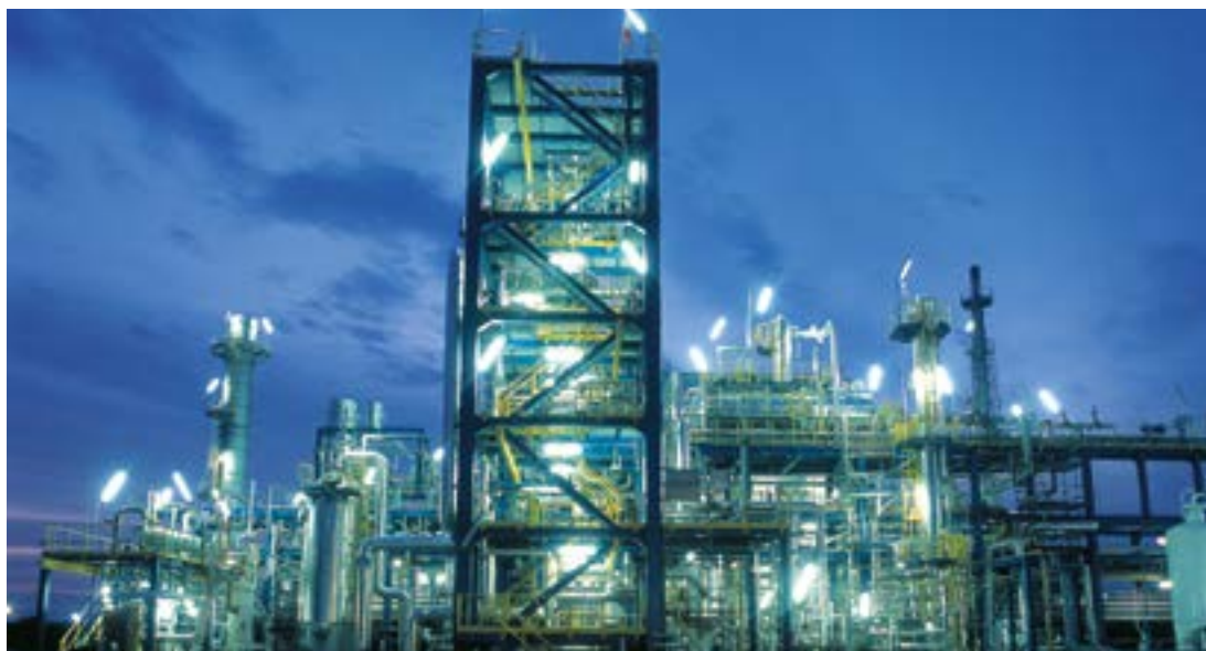
Figure 2.1: Air Liquide hydrogen production plant (source: AIR LIQUIDE Deutschland GmbH)
