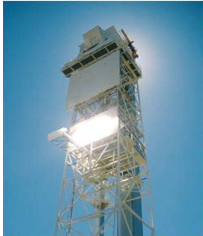
Figure 2.8: Pilot installation for solar/thermochemical production of hydrogen on a solar tower (source: DLR)
