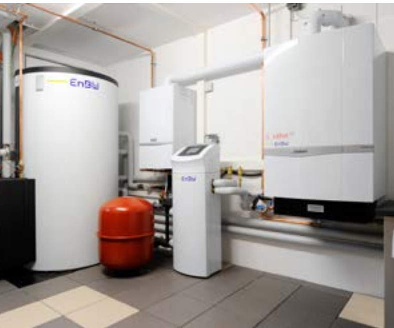
Figure 4.5: Vaillant field-testing system for the Germany-wide Callux practical-testing programme (source: Vaillant GmbH)
